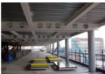
*Paires de poutres alvéolaires*
